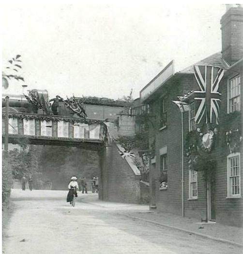
Station Road railway bridge in about 1905
