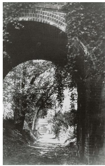
Bridge over Waddling Lane
