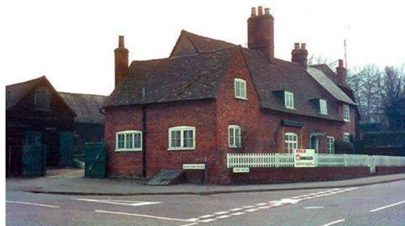
Town Farm shortly before demolition
