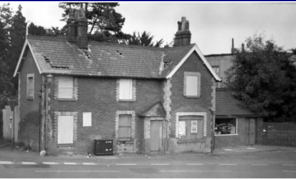
Wheathampstead Station before demolition to make way for the by-pass
