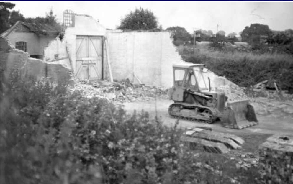
Demolition of building in Station Yard
