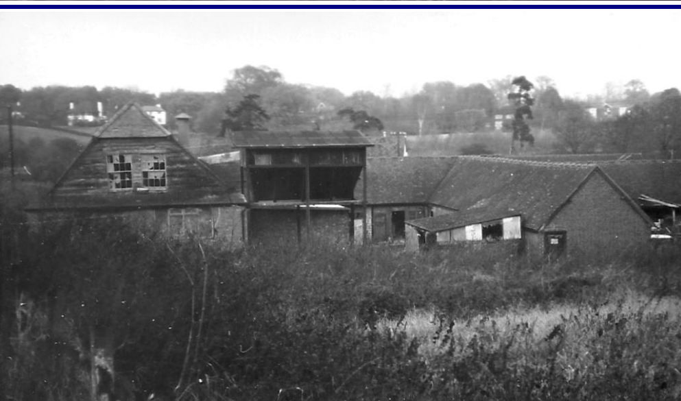
Another view of Bury Farm before demolition
