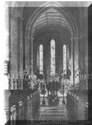
Interior of St Helen's Church
