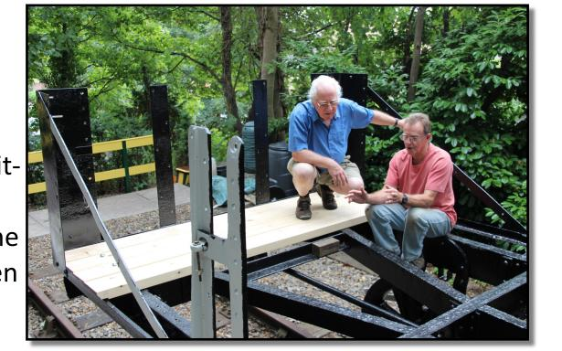
coats, one undercoat and two topcoats. The lettering is protected with a coat of lacquer. The planks, most of which were paid for by our generous sponsors, are fitted to the frame using more than 250 bolts.
